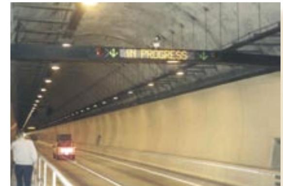
Figure 4: Variable Message Sign in an American tunnel
